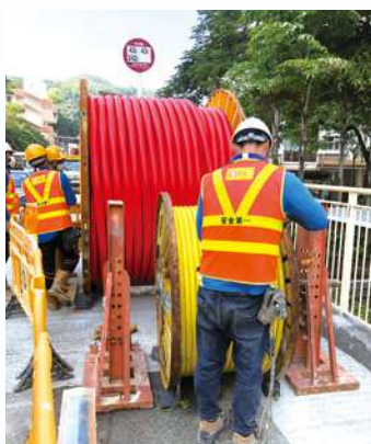
Cable Trenching And Installation Works
